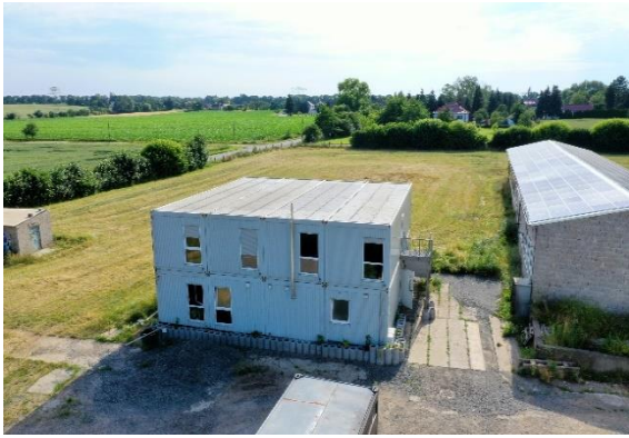
Move to new location: Container office on site (January)
